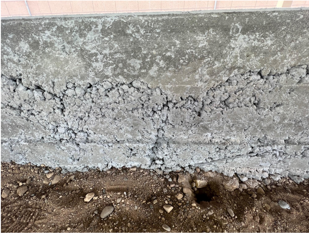
Thickened concrete slab edge. Image courtesy of APEX (08.23.2023)
