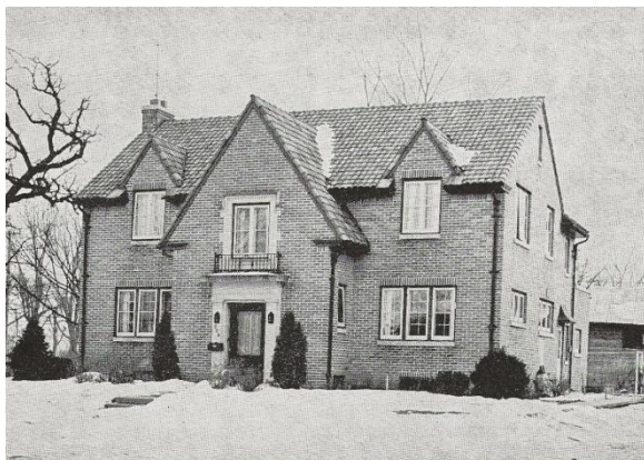
The Present Rectory Build in 1933
